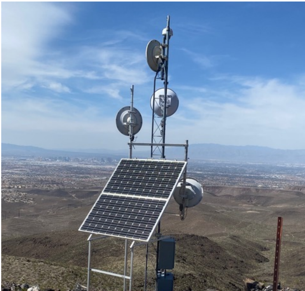
Migration to 11GHz point-to-point radio in Henderson NV
