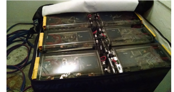
Qty 6 Genasun LiFePO 4 batteries installed at a TA-AK site in protective bag
