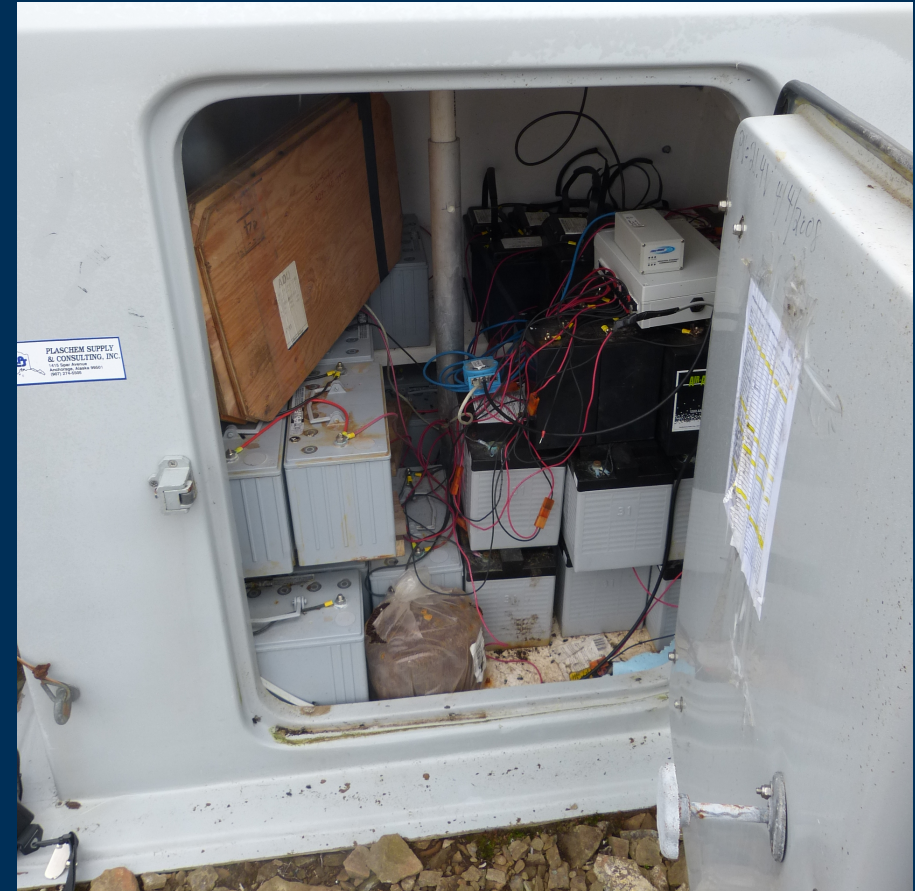
2 separate power systems in 1 hut (poor integration)
