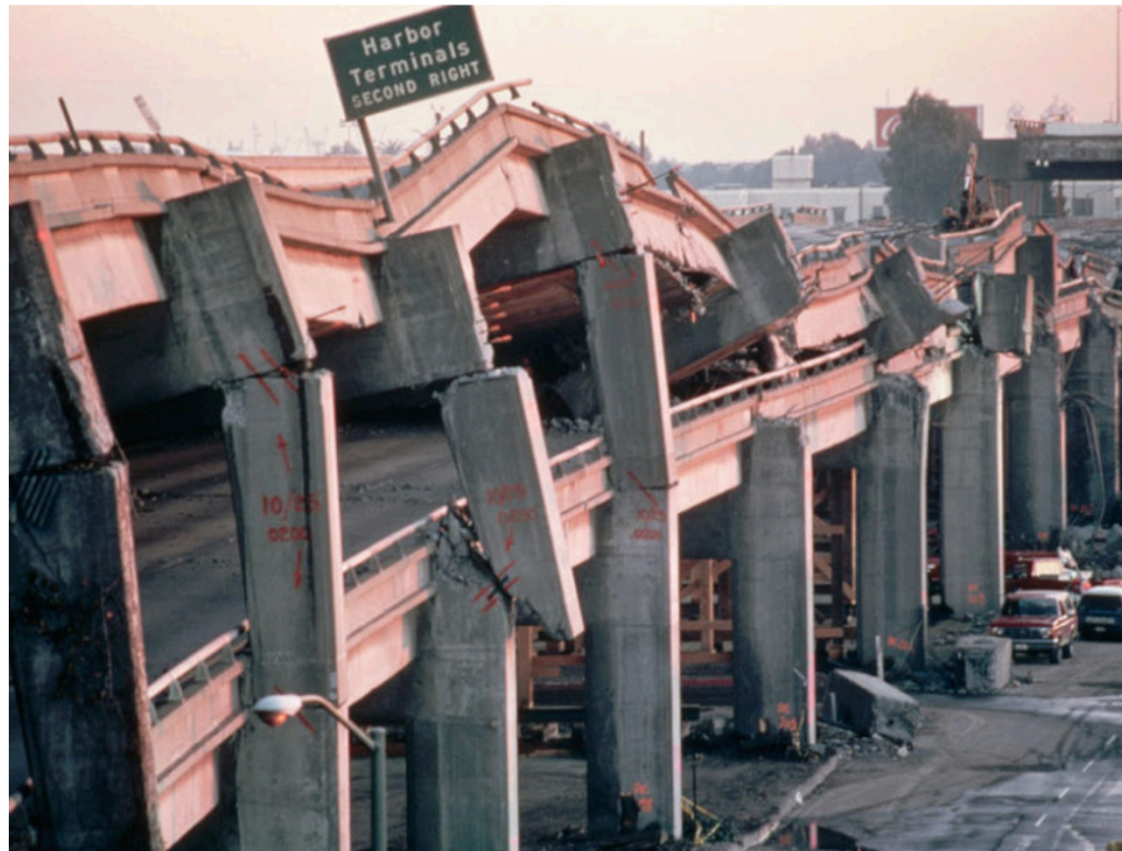
The Cypress Freeway collapsed from the Loma Prieta earthquake in the San Francisco Bay Area in 1989, killing 42 people. Credit: Jim Sugar/Corbis Historical/Corbis via Getty Images
